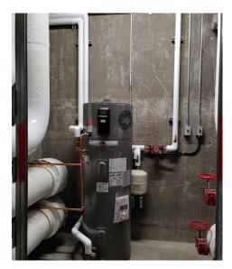
Figure 2: Heat Pump Hybrid Domestic Hot Water Heater
