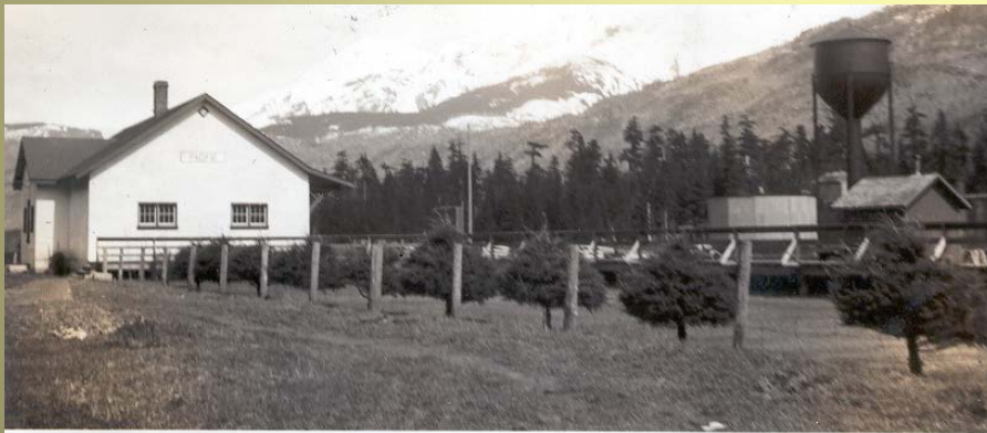
Pacific second GTP Station Courtesy of "The McCubbins" website
